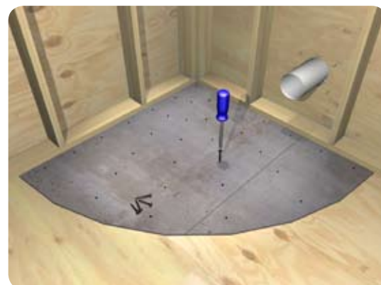
Figure 10 - Masonry Board Installation
