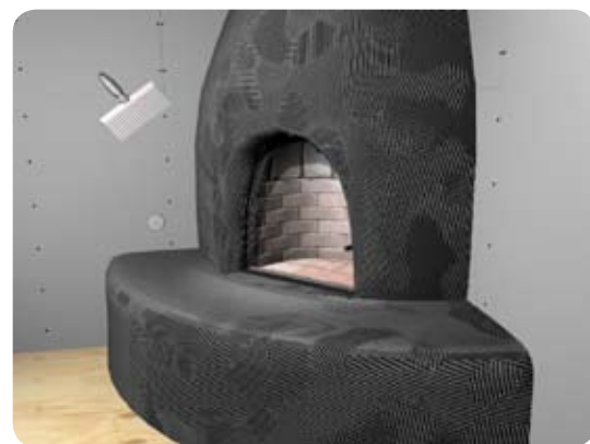
Figure 35 - Scratch Coat
