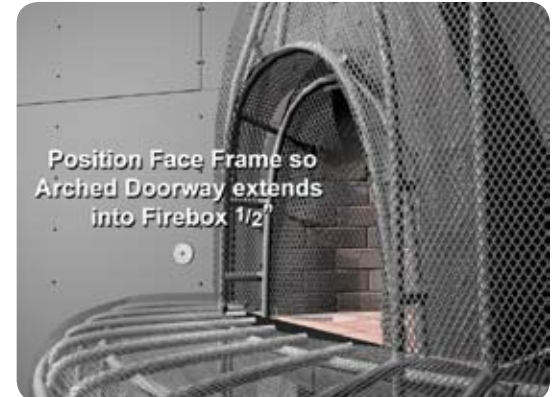
Figure 30 - Face Frame in Place
