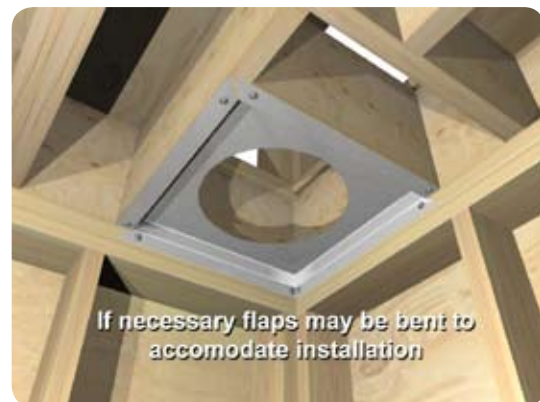
Figure 24 - Ceiling Firestop Spacer
