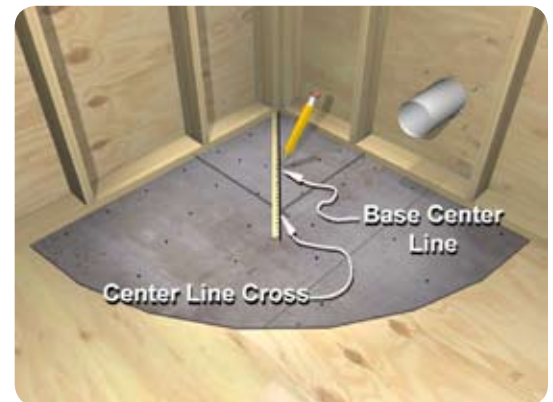
Figure 12 - Base Center Line
